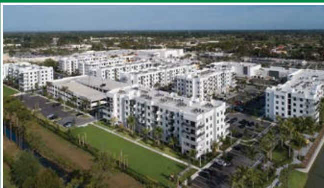
TWO PARKING STRUCTURES
